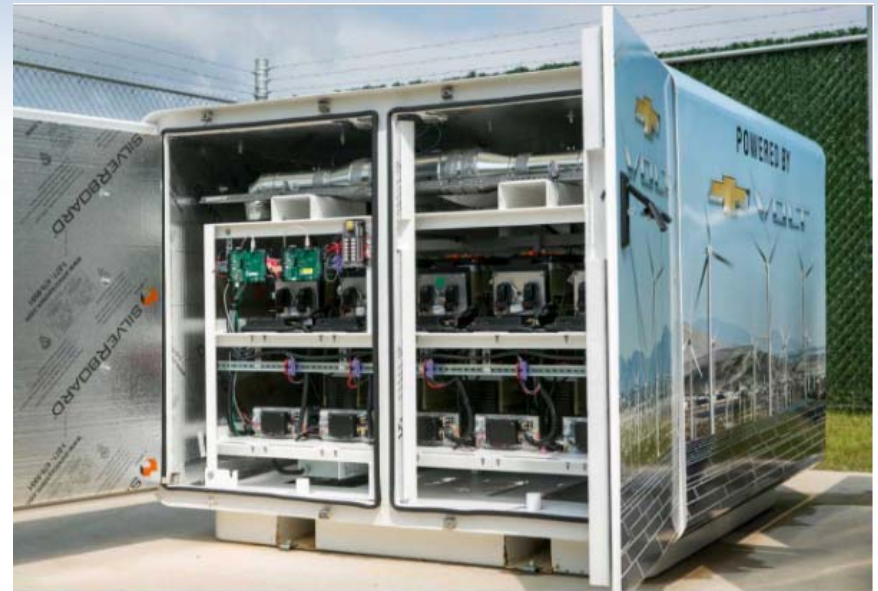
Used Chevy Volt Batteries Help New GM IT Building Use Solar And Wind Power. Via GM and Joe Romm
